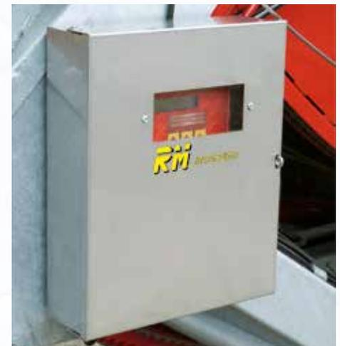
Protection stainless steel box for RainMaster 2.6 programmer
